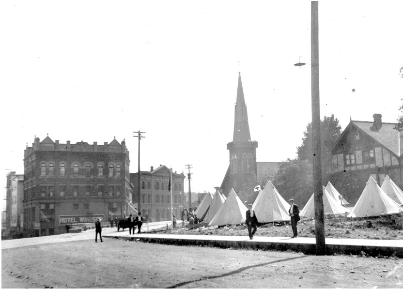
Figure 8. Looking south along Front Street, Nanaimo, August 1913, showing the camp of the 72nd Regiment, Seaforth Highlanders of Canada, on the grounds of Nanaimo Court House, with St. Paul's Anglican Church behind and the Hotel Windsor at left. Photographer unknown. Source: Image A-00980 courtesy of Royal British Columbia Museum, B.C.A.
